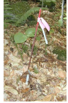
Marking a site corner with painted rebar and flagging tape
